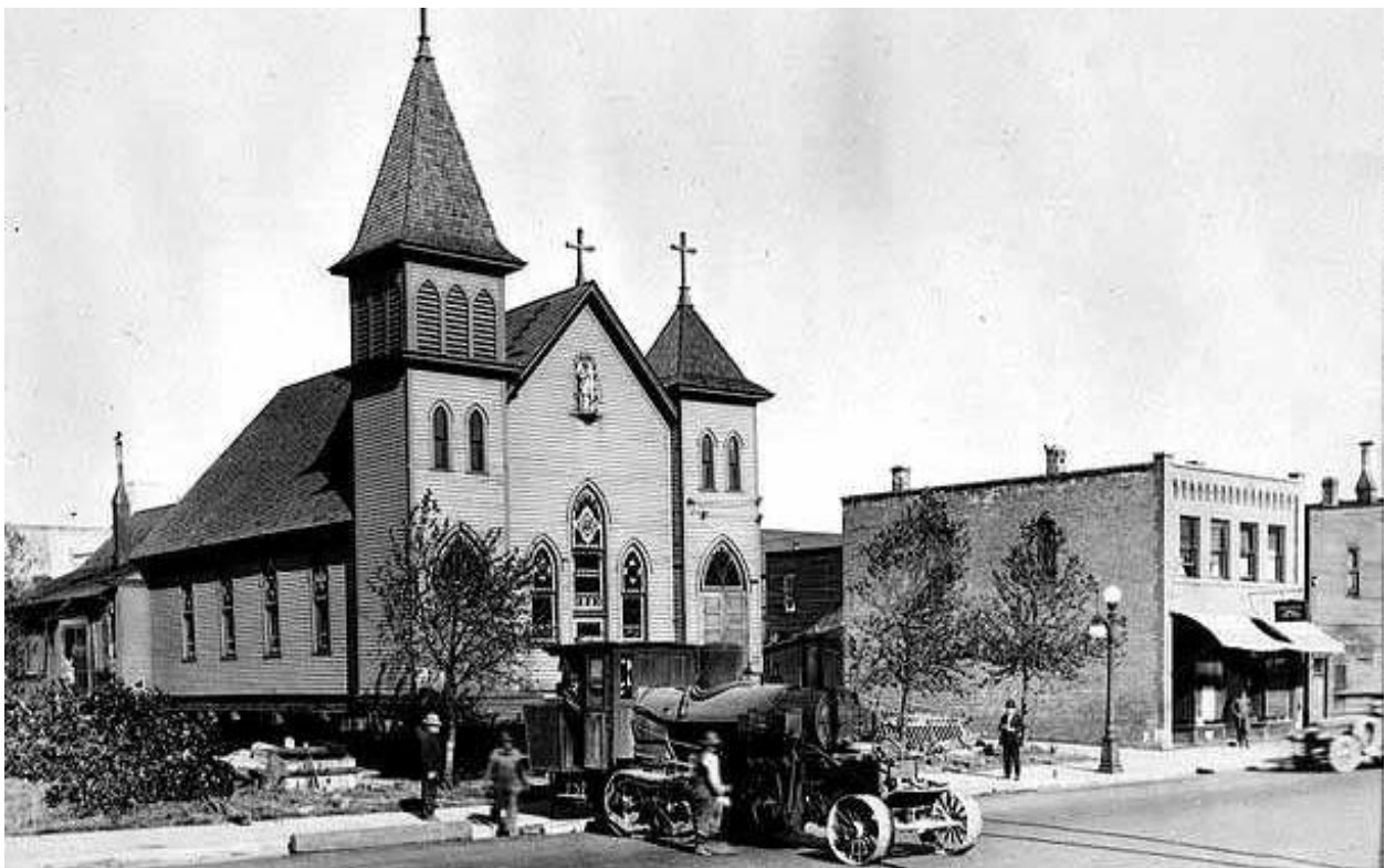
Figure 3. Moving a church from the old to new townsite of Hibbing, 1920
